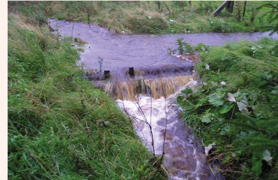
Figure 3 Upstream bund diverting flow into field.
