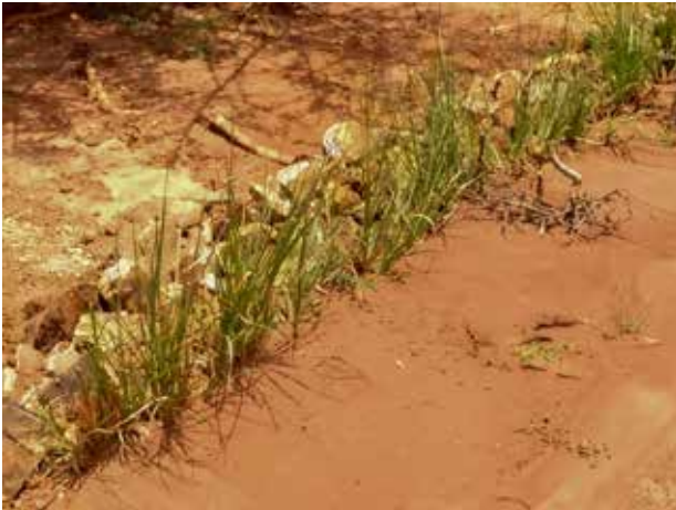
Fig. 13: Rock check dams and lines of vetiver grass planted to reduce the speed of surface run off. Vetiver grass planted along a contour line to make a permanent biological barrier.
